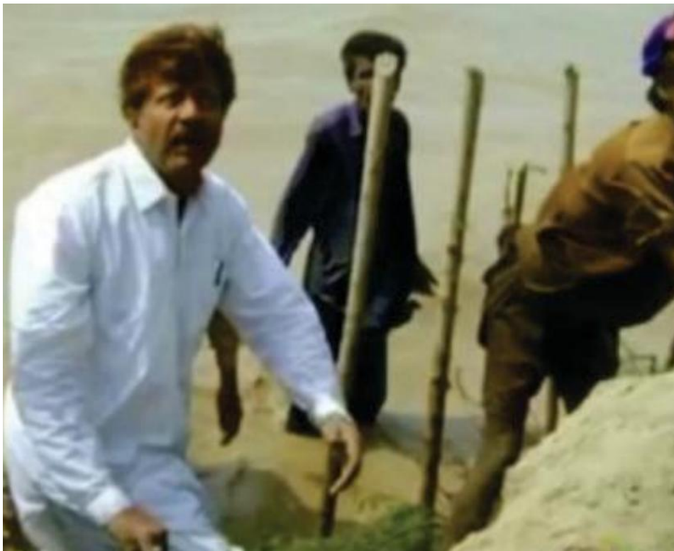
MNA Syed Shafqat Hussain Shah Shirazi Personally Engaged in Repairing a Flood Protection Embankment
